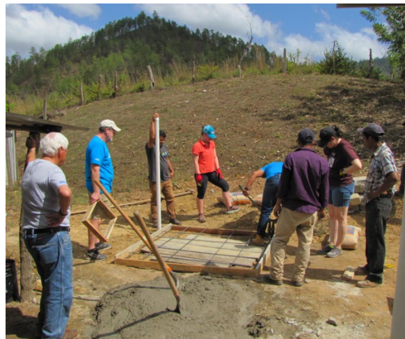
And constructing the septic tanks
