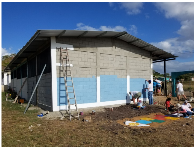
Painting the new school addition
