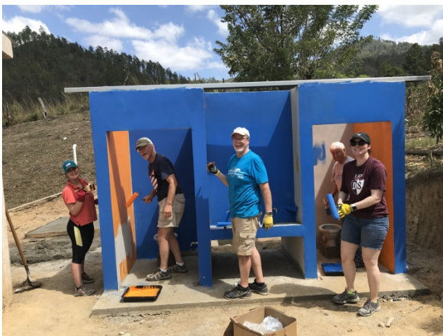
Team Members Painting the Latrines .....
